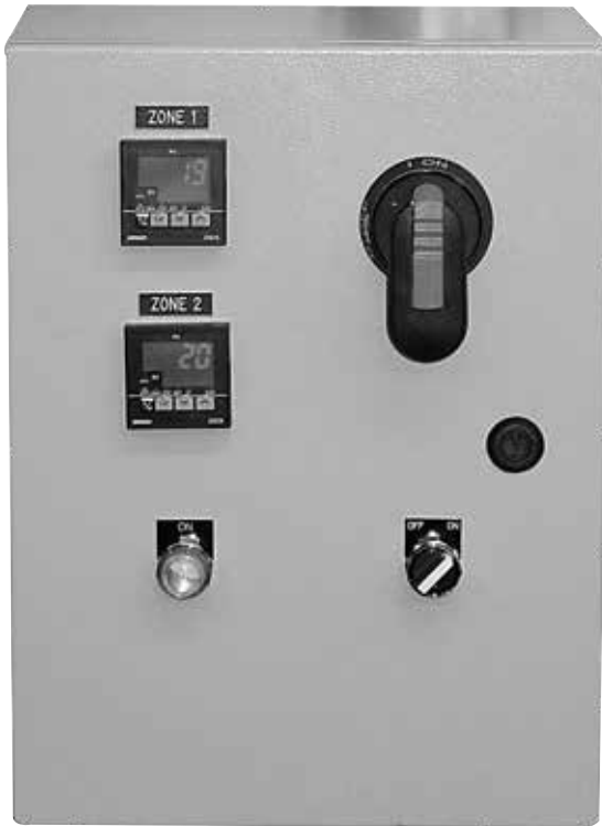
Front of Control Panel
