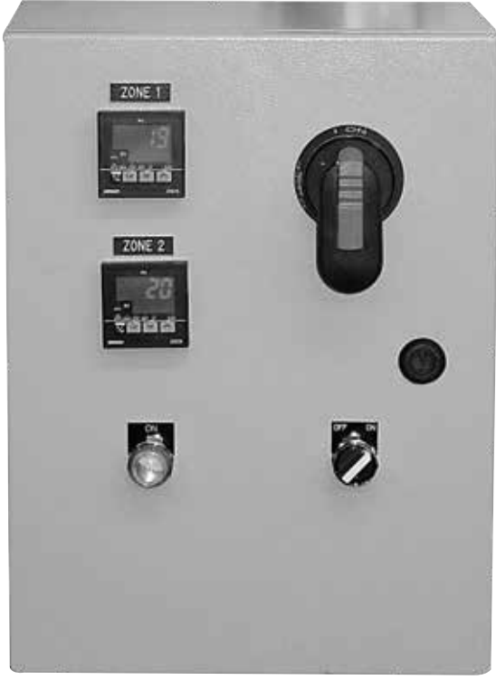
Front of Control Panel
